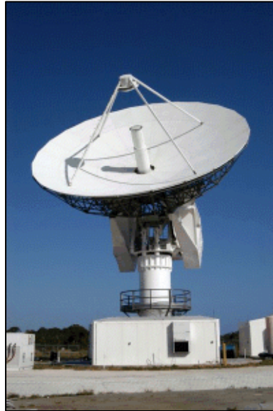
An example of a parabolic antenna with a secondary (or sub) reflector
